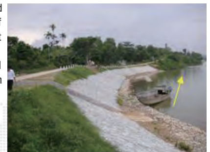
Test Construction of Riverbank Erosion Protection Works
