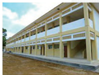
Earthquake Resilient School in Indonesia
