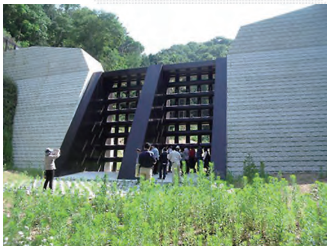
Permeable Sand Control Dam under Rokko Sabo Office, Kinki Regional Development Bureau, MLIT
