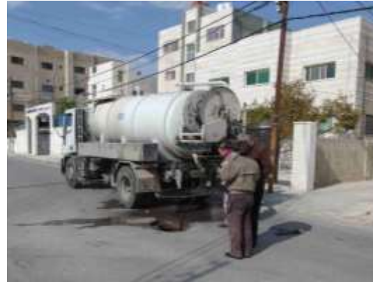
Flushing of clogged sewers
