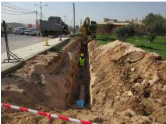
Construction of urgent backbone pipelines for tangible service improvement
