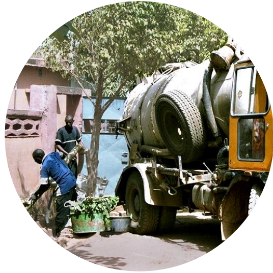
Photo: mechanical emptying in Mali. Credit: Eawag-Sandec
