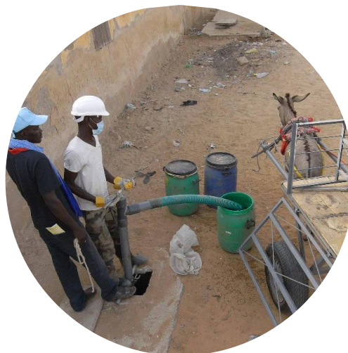
Photo: manual desludging with a Gulper in Rosso. Credit: EnHaut
