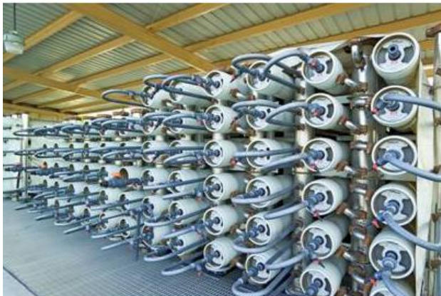
RO for Industrial Boilers (1x and 2x)
