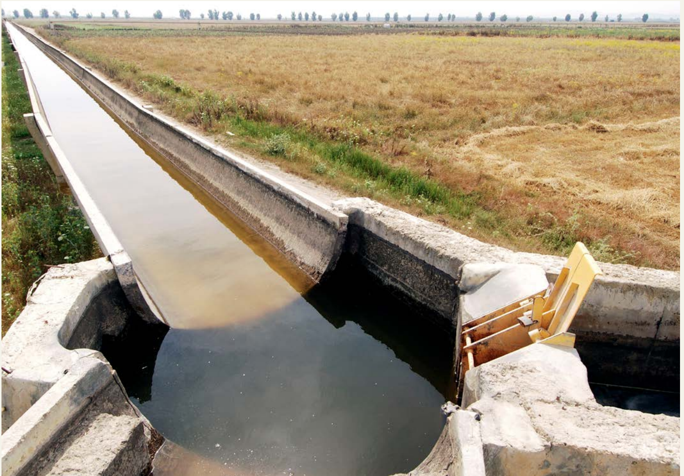
Irrigation canal, Morocco.
