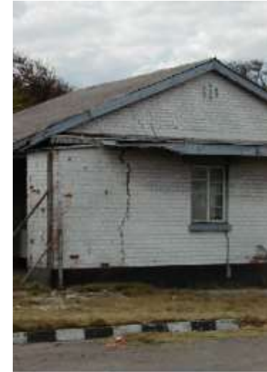
Cracking due to tremors caused by underground blasting and in some cases subsidence
