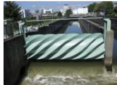
Small Hydro Power
