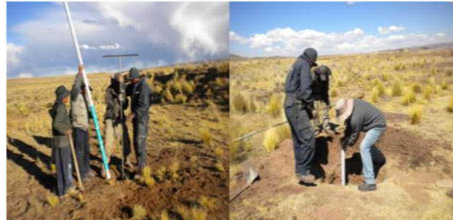
'Installation of piezometers for hydrogeological study' - Bolivia
