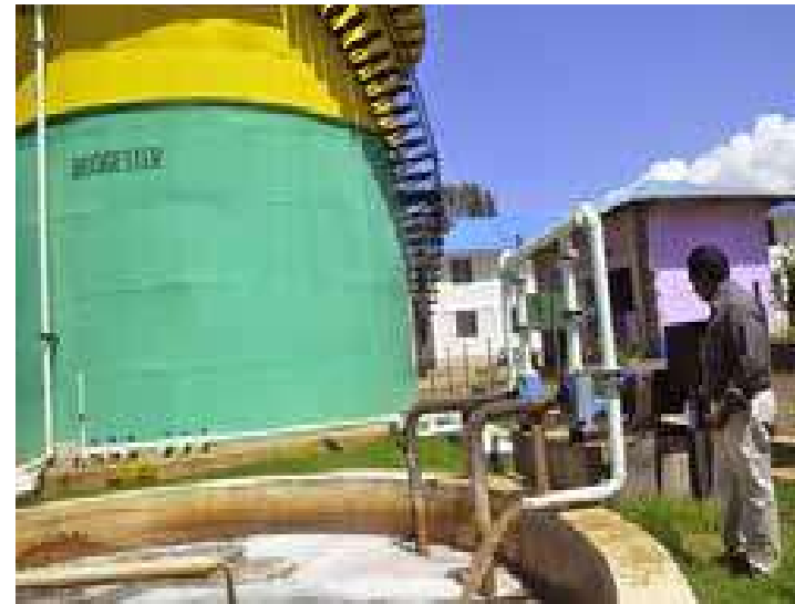
Wastewater treatment system installed that purifies wastewater and generates biogas at Banana Investments - Tanzania
