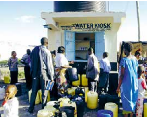
Utility operated water kiosk, Kenya
