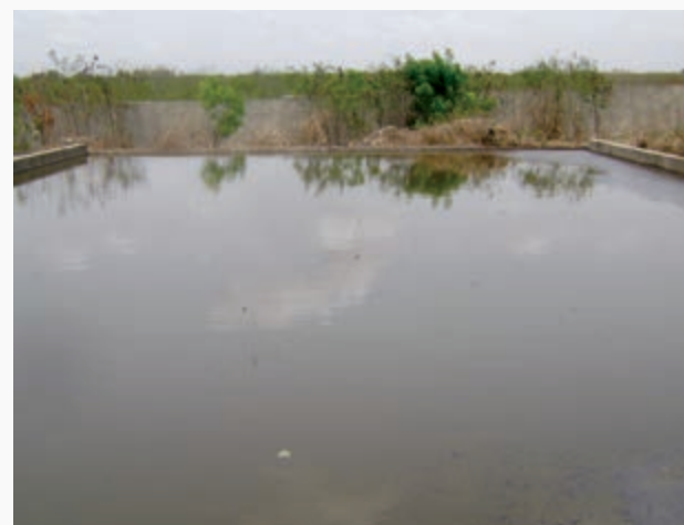
b. Fresh FS on the drying bed (on day 1).
