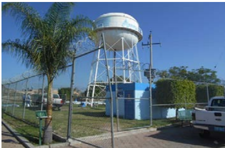
Elevated tank -SAPAF
