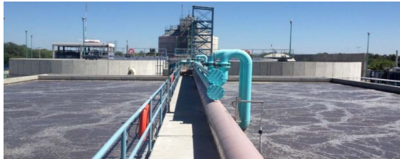
“San Jeronimo” WWTP
