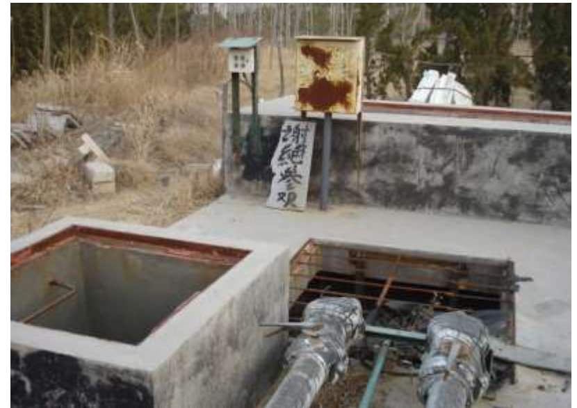
semi-decentralized WWTP with a capacity of 400 m 3 /d, operating since 2013
