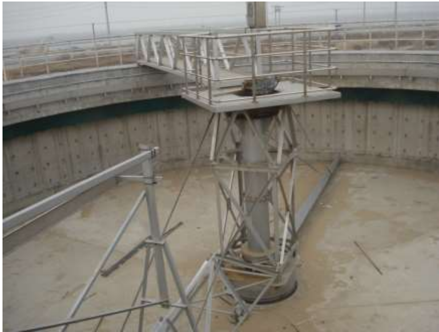
WWTP with a capacity of 10,000 m 3 /d, 15 km from center of development area, not operating
