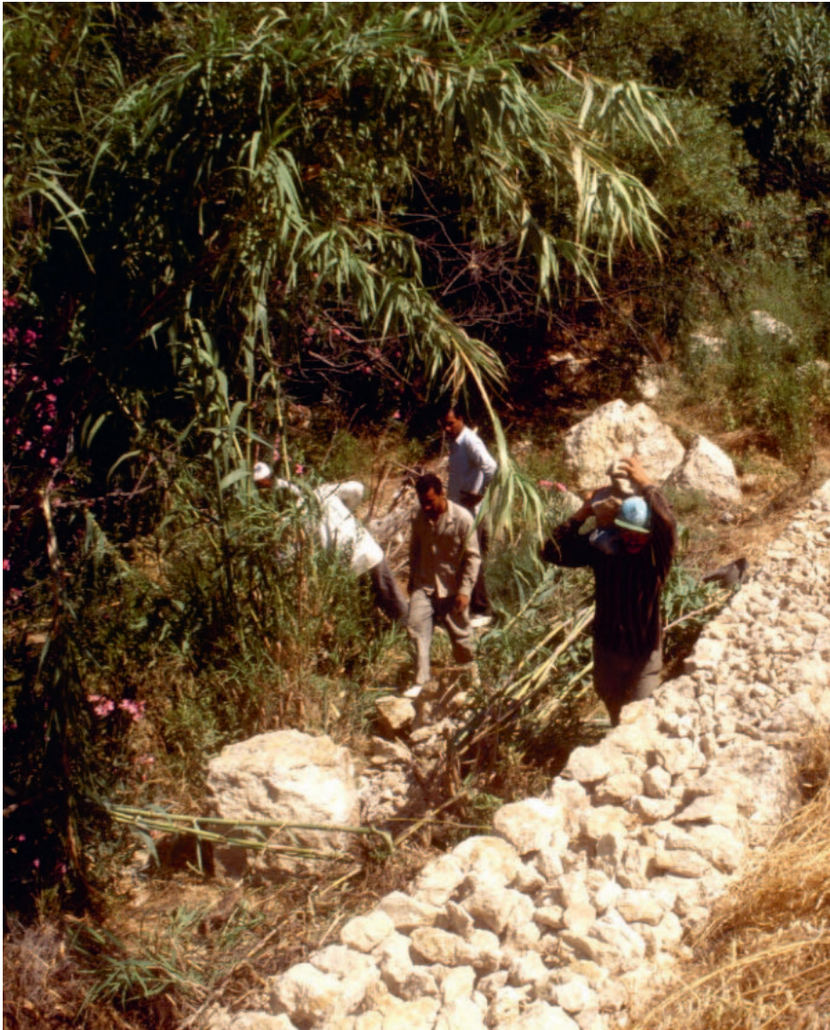
Jordan. Construction of a dry wall to protect cultivated land from water erosion. © FAO/Roberto Faidutti.
