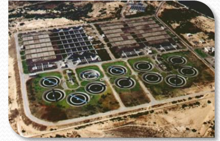
secondary treatment – 130 MCM/Y effluent
